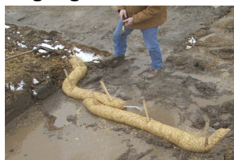
Overlap Sections 6 “ (min)
