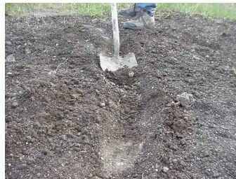
Dig Shallow Trench
